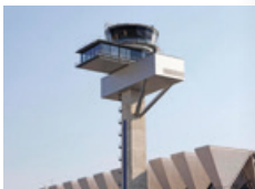
③ New air traffic control tower
